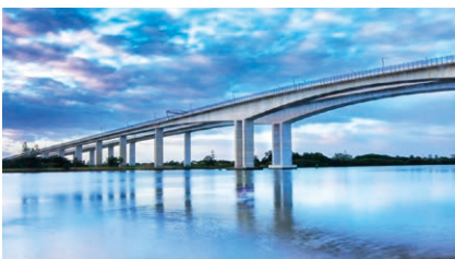
Monitor infrastructural deterioration in bridges
